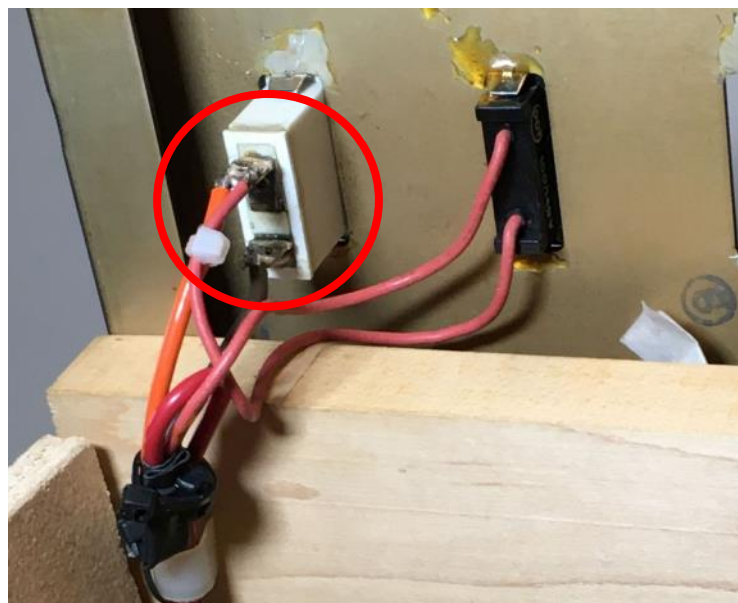
Exposed wiring at on-off switches is a common hazard
